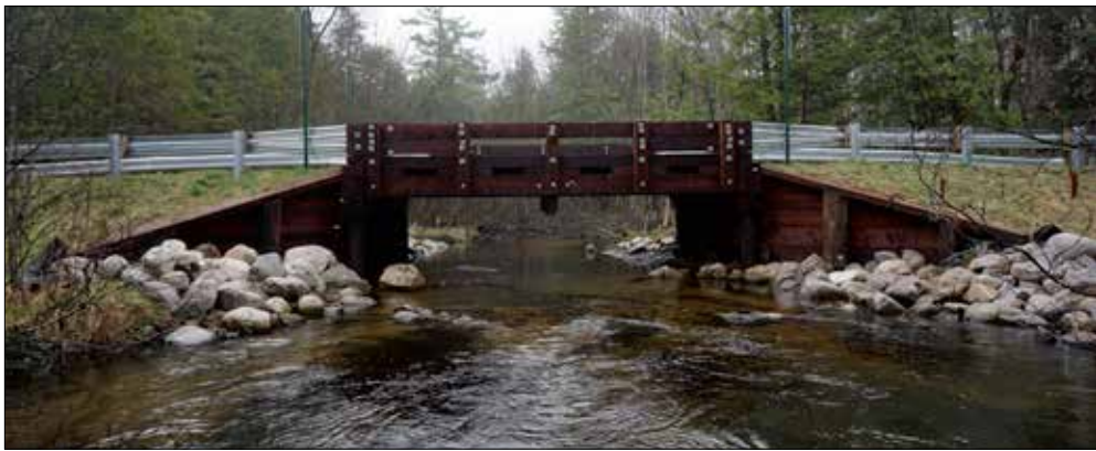
Bridge work before (top) and after (bottom). Photos courtesy of Conservation Resource Alliance.
